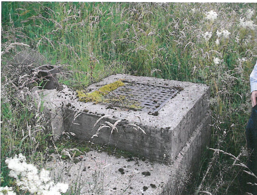
Photo 10 – Manhole on scour valve
